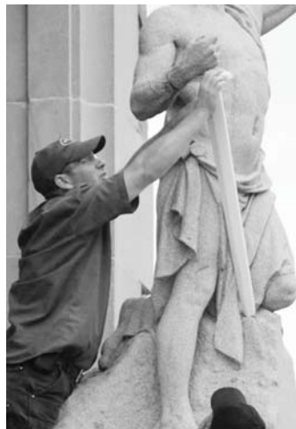
Rearming a warrior: the Styrofoam sword template is checked for fit on the Malvern statue. Right, the original brochure.
