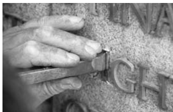
Lost art: replacement letters in lead were pinned in place and carved one at a time by hand. Below, the memorial's base was repaired to make it stable.
